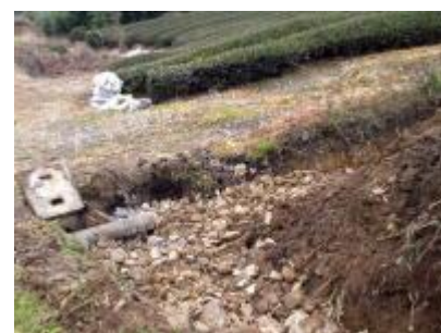
Improving water facilities at the tea farm
