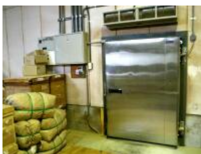
Cold storage chamber
